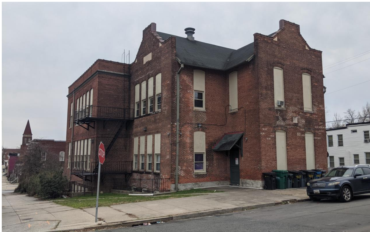
Image 6: The Gorsuch Avenue and Tyler Street elevations in January 2021.
